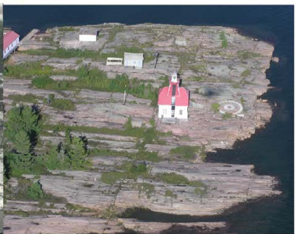
Snug Island Lighthouse from 500 feet
