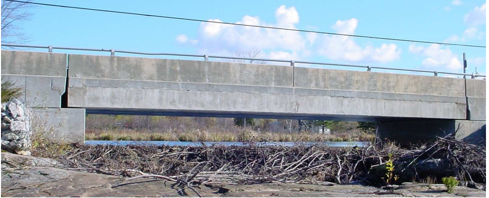
Beaver Dam Debris at Dillon Bridge, Earl Milligan
